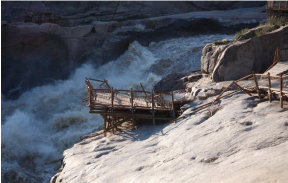
Augrabies storm damage of January 2011 still visible in May 2011
